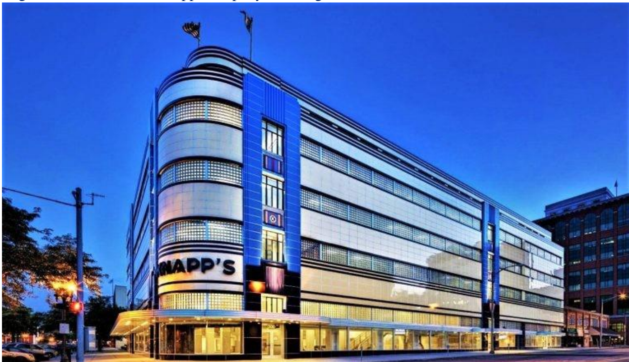
Figura 1: Edifício J.W. Knapp Company Building.
